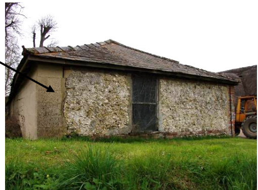
Figure 10: Shed west of Peasmore House. The south elevation has been constructed of 'wychert'.
