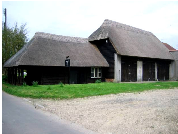
Figure 13: Barn at Manor Farm
