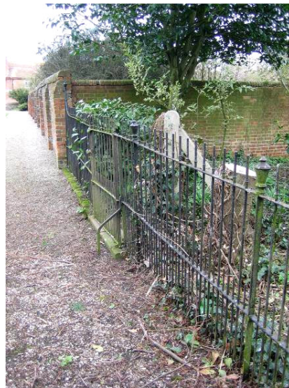
Figure 33: Cast iron railing with decorative urn finials along the southern boundary of the churchyard
