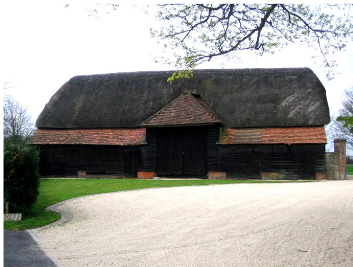
Figure 38: Mixed use of thatch and plain tiles at the Grade II listed Prince's Farm.
