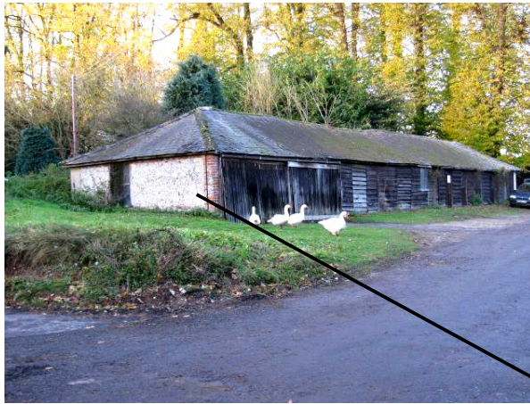
Figure 10: Shed west of Peasmore House. The south elevation has been constructed of 'wychert'.
