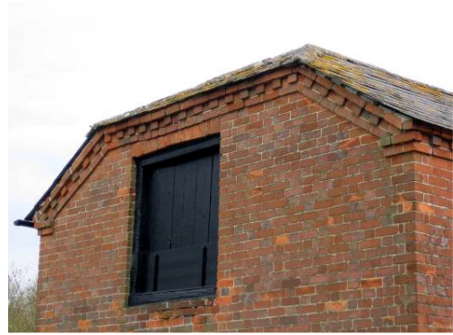
Figure 24: Eaves and verge details on brick buildings are articulated by brick dentils
