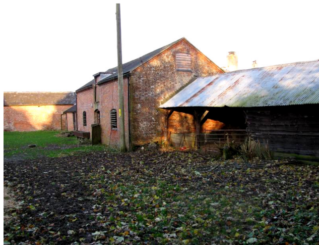
Figure 11: Stables west of Peasmore House. The building running at right angles to the stable is the Coach House.
