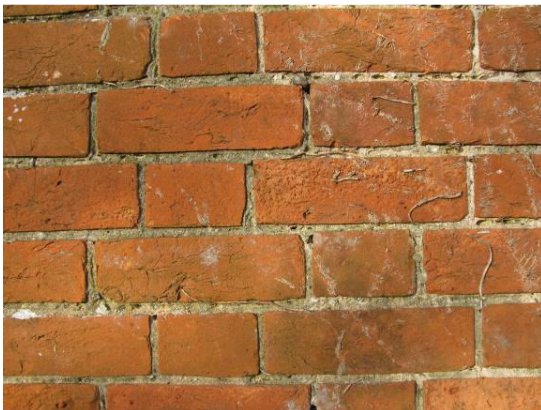
Figure 19: Orange-red brick set in lime mortar at Princes Farm
