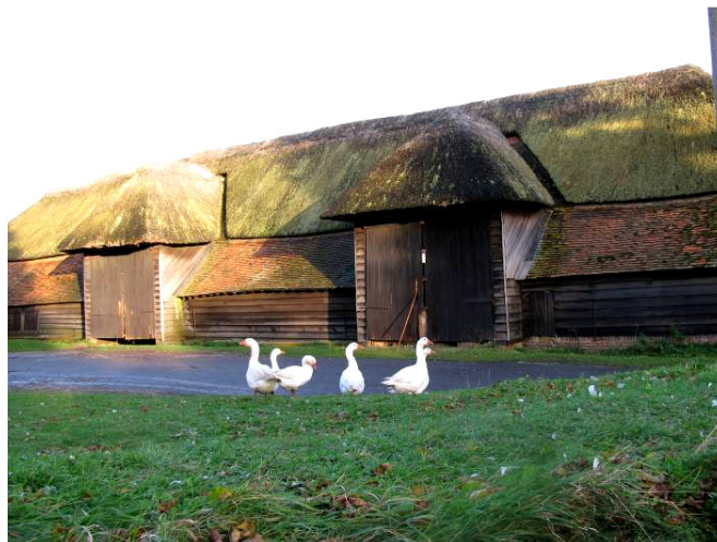
Figure 28: Barn west of Peasmore House (Early 17 th century, Grade II listed). The main roof is thatched but the aisles are tiled.
