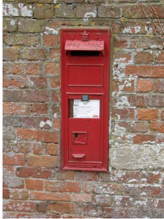
Figure 42: Wall-mounted post box inserted into a boundary wall
