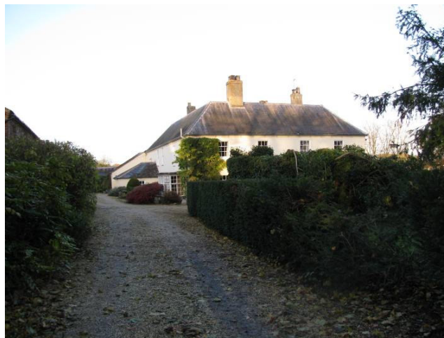
Figure 44: Peasemore House, Chieveley Road
