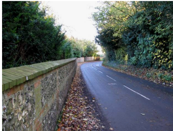
Figure 30: Flint and brick boundary wall of Peasemore House lines the road providing a horizontal emphasis.
