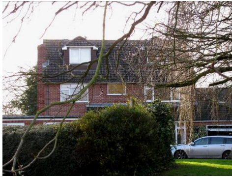
Figure 51: Dormers set high into the roof, concrete pantiles and inappropriate windows do not reflect the local vernacular.
