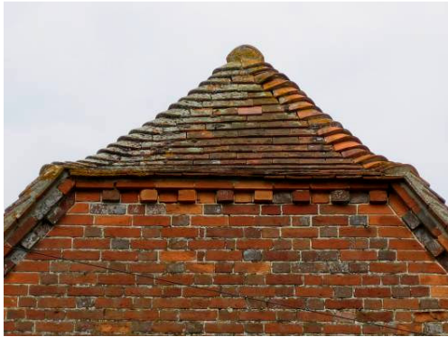
Figure 24: Eaves and verge details on brick buildings are articulated by brick dentils
