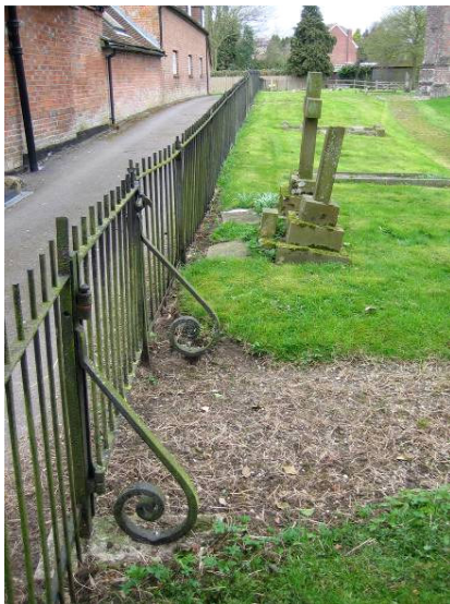
Figure 32: Railings and gate, supported by elegant scrolls, along the western boundary of the churchyard.
