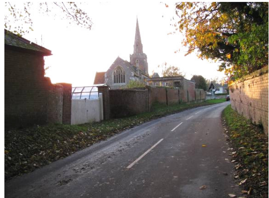
Figure 5: Emerging from the enclosed brick-walled lane (known as Chieveley Road) lined with towering trees, one gains a first glimpse of the church and starts to sense a feeling of openness.
