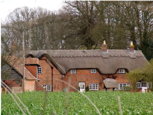
Figure 39: West elevation of Princes Cottage Farm
