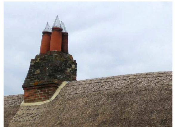
Figure 26: The chimney punctuates the flush ridge thatching of Paxmere House.
