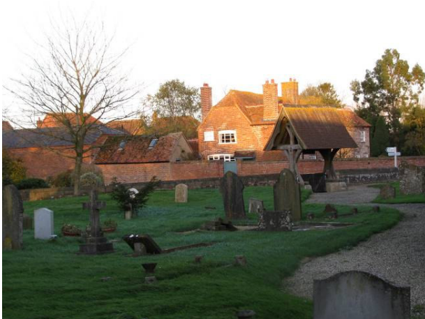
Figure 25: Brick chimneys at Manor Farm add interest to the roof
