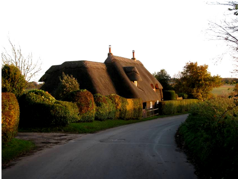
Figure 22: The dramatic roof of Elm Tree Cottage (19 th Century), Chieveley Road
