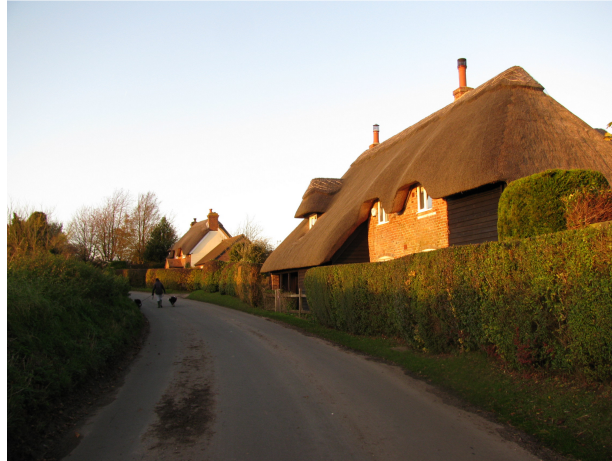
Figure 18: Elm Tree Cottage (in the foreground) and Bramble Cottage
